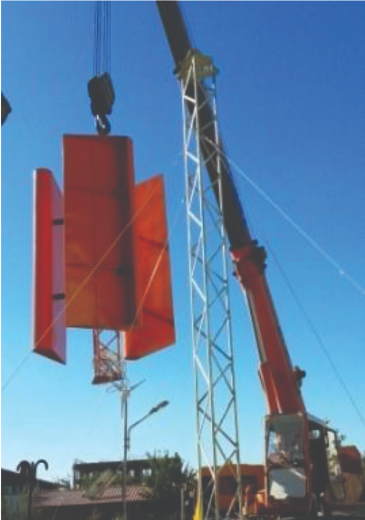
Figure 13: Crane lifting the top of the wind turbine.
